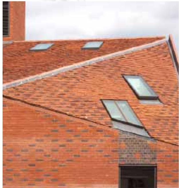
Fourteen neo rooflights in two sizes complement the clean unelaborated, mostly recessed window openings, while providing high levels of light and ventilation for the classroom accommodation on the second floor. In order to control solar gain and reduce noise pollution, a combination of Pilkington Suncool™ and Optiphon glazing was specified. The bespoke trapezoidal rooflight in the same style as neo, but with glazing bar illuminates the classroom space below.
