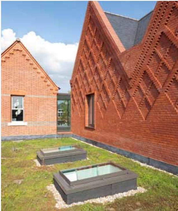
Natural light and ventilation are provided by a total of eight low-profile Plateau rooflights with electric actuation. The lower level sedum roof features two Bespoke Plateau Rooflights (1.5m x 0.9m).
